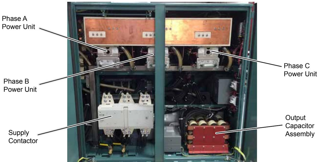
FIGURE 43 - CENTER AND RIGHT SECTION OF DRIVE CABINET HYP1278A
